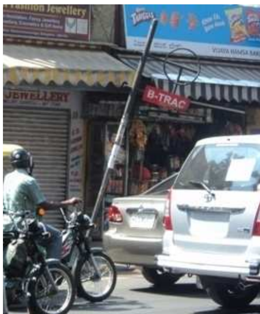
Figure 3.16: Traffic Signs not properly made and erected
